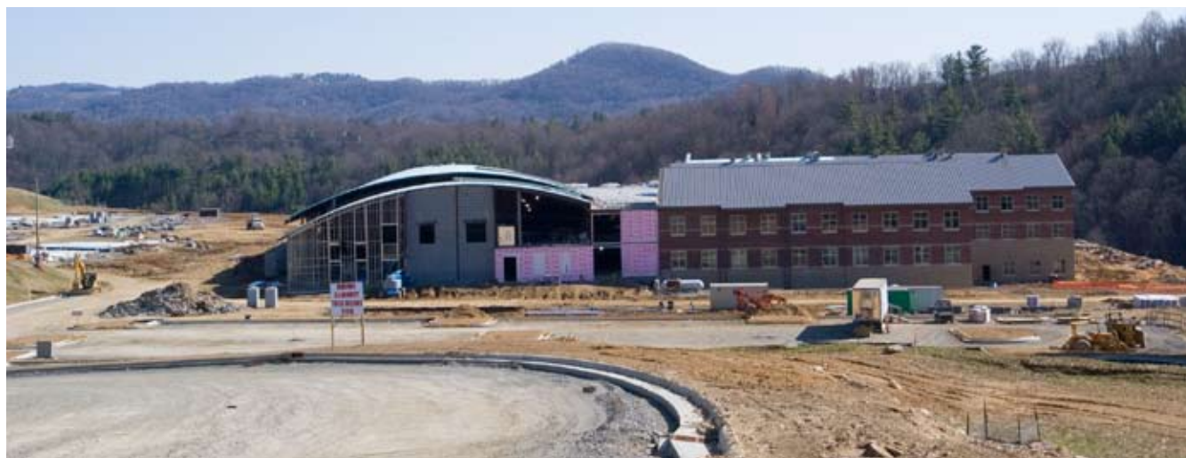
Watauga High School under construction, March 2009
