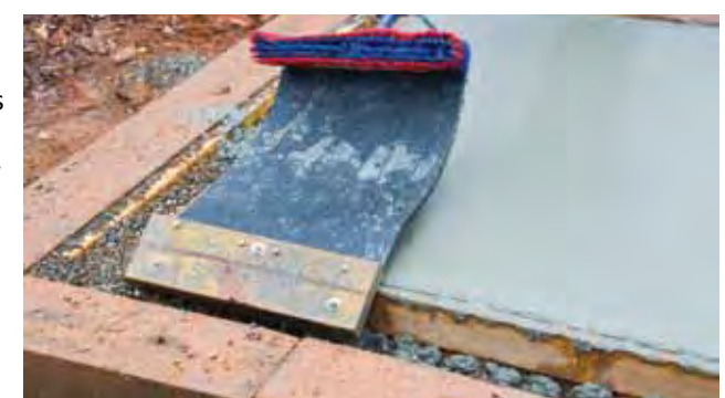
The texture tool: broom, a few screws, washers, a 2x6, and AstroTurf mat.
