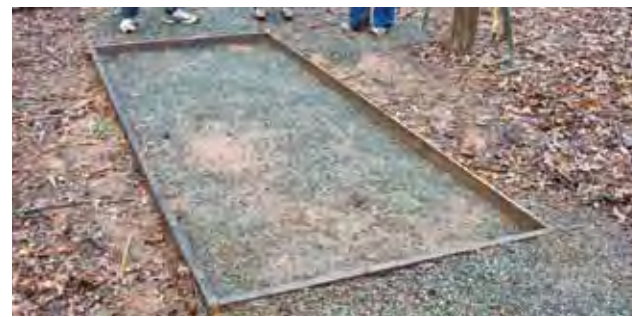
Frame is ready for concrete.
