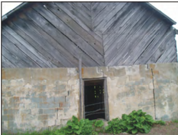
Photo Five: View of structure number 7, barn, built in the 1930's.
