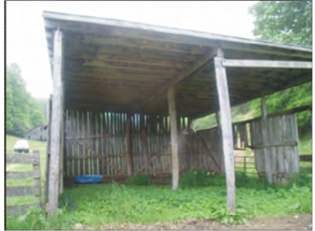
Photo Seven: View of structure number 6, pole shed, built in 1995.
