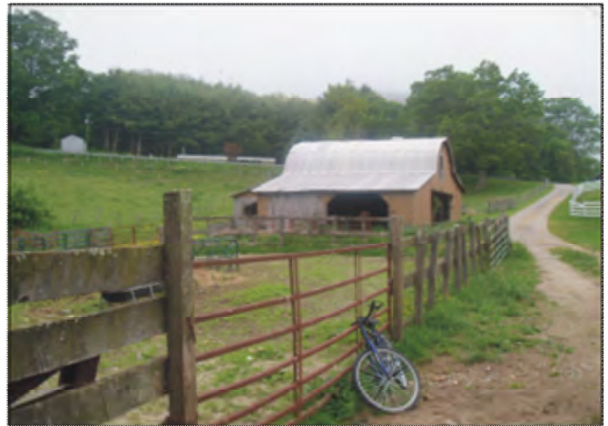
Photo Two: View of Structure 2, barn, built in the 1940's.
