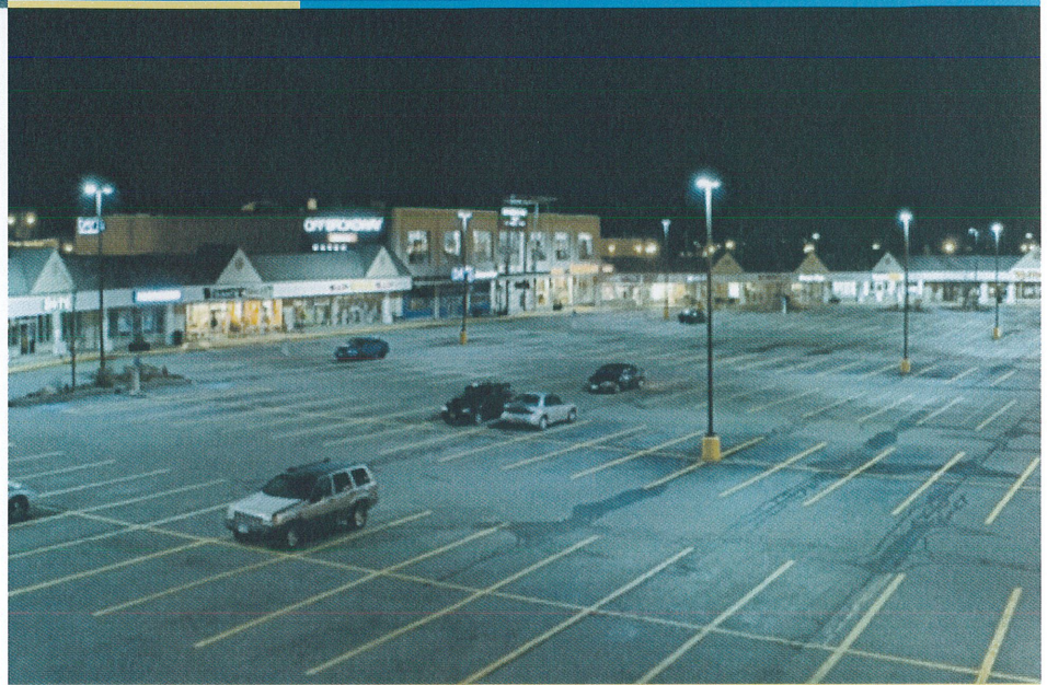
Parking lot after installation of LED luminaires
