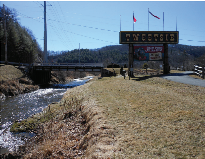
Existing Portion of the Greenway and the Middle Fork Creek
