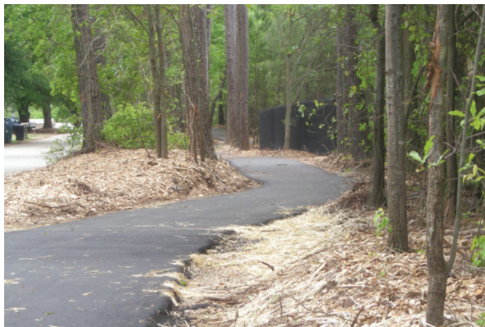
Wadsworth Trail - Spartanburg County : After Construction
