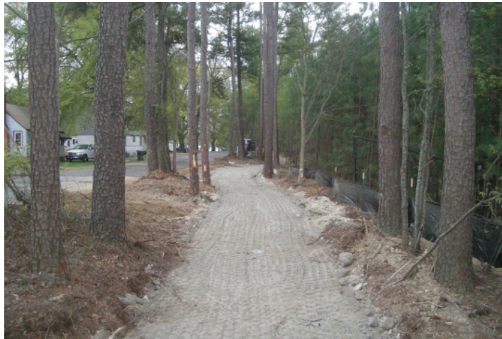
Wadsworth Trail - Spartanburg County : During Construction
