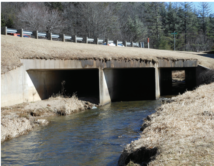
Close Up View of the Existing Culvert Crossing
