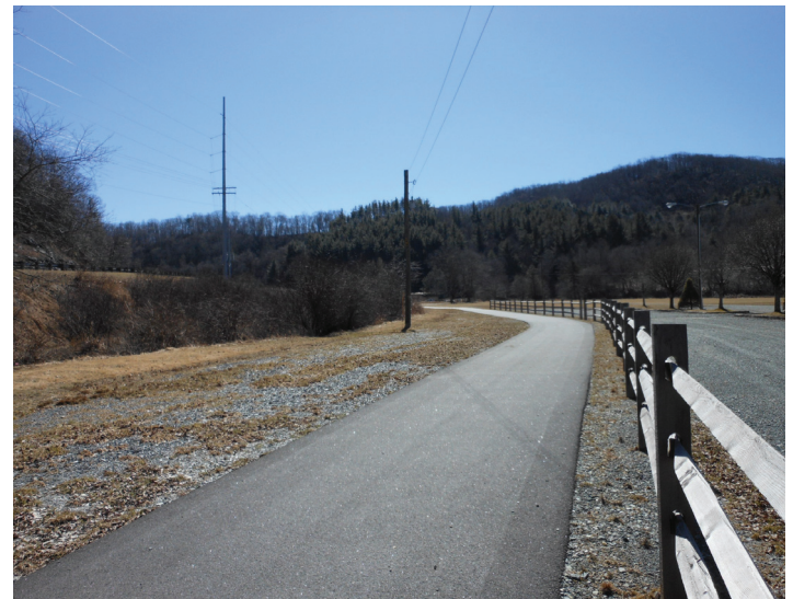
Existing Trail Portion with Split Rail Fencing
