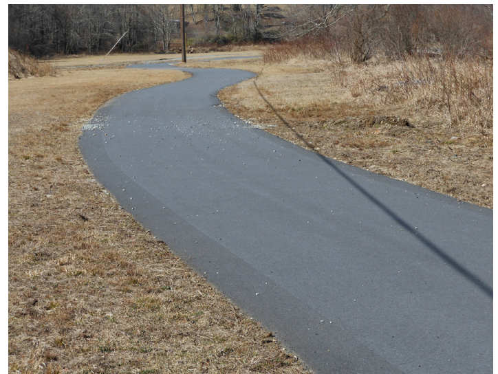
Portion of the Existing Trail on a Curve
