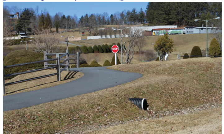
Existing Trail Portion with Stormwater Pipe
