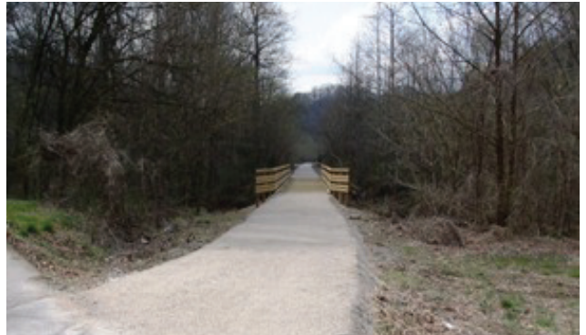
After Construction Trail View
