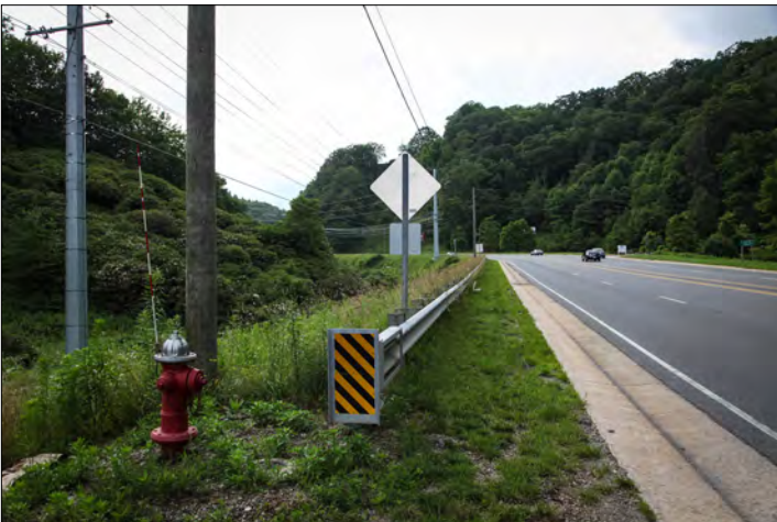
ROUTE A WOULD UTILIZE THE NCDOT RIGHT-OF-WAY FOR APPROXIMATELY 2,900 LINEAR FEET.
