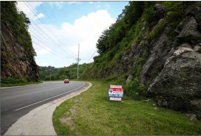
ROUTE A WOULD PARALLEL A MAJOR ROCK OUTCROPPING LOCATED NEAR ROARING RIVER DRIVE.
