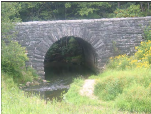
PHOTO OF CULVERT HEADWALL
