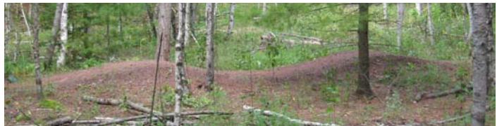
Deno’s work creating a classic roller, paying special attention to height/crest spacing ratio to ensure rideable flow at varying speeds.
