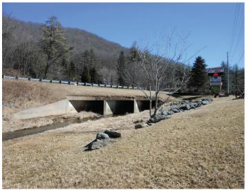
Existing Culvert Crossing - The proposed trail will go under existing US 321 inside this culvert.
