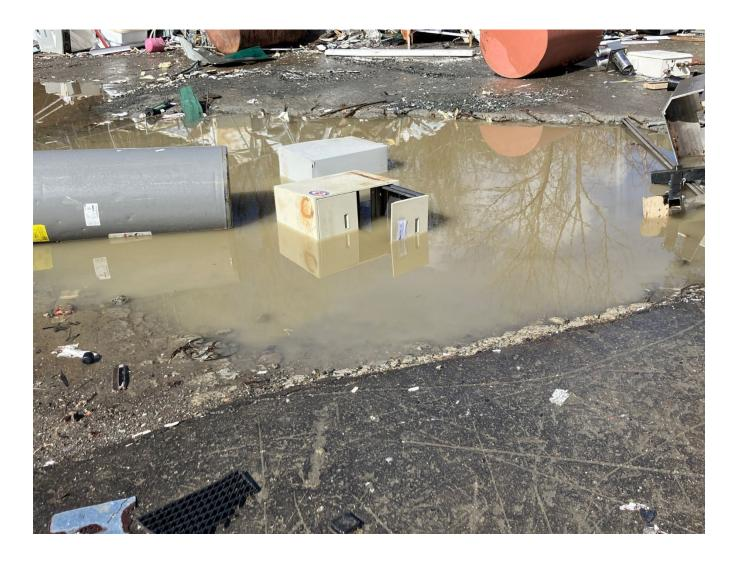
ABOVE: One of two areas in the current scrap metal pad that has degraded enough to hold water. Exposed rebar is also visible along the top of the 'lake'.
